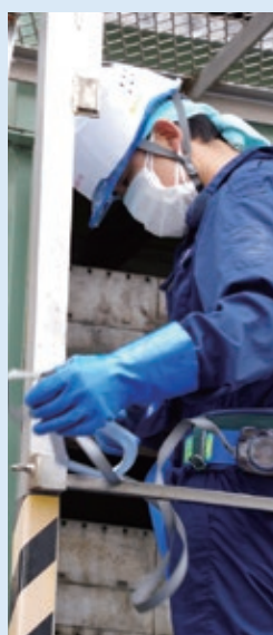
Left: Replacing the activated charcoal used in the deodorizing equipment Right: Employees always wear safety harnesses to protect their lives when performing operations in high places.
