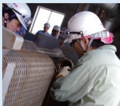
Ensuring stable production by taking apart a heat exchanger and washing each section by hand
