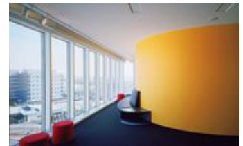
Thermal storage tank Less expensive nighttime power is used to chill water in the tank, which is then utilized to cool the office during the day
