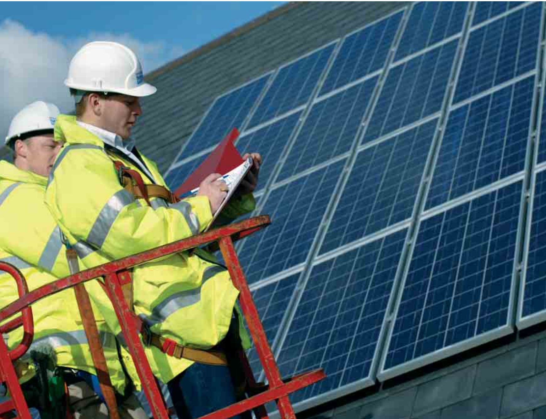
Photovoltaic cells, which convert solar light into electricity, cover an area of 30 sqm at the Cyan Building, Rotherham.
