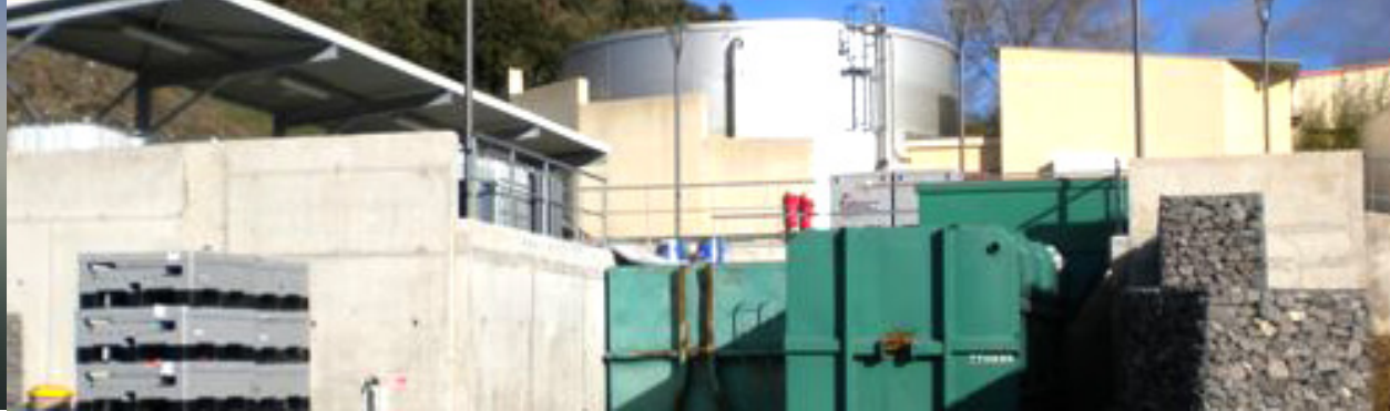
The waste-sorting platform at the Lagorce factory
