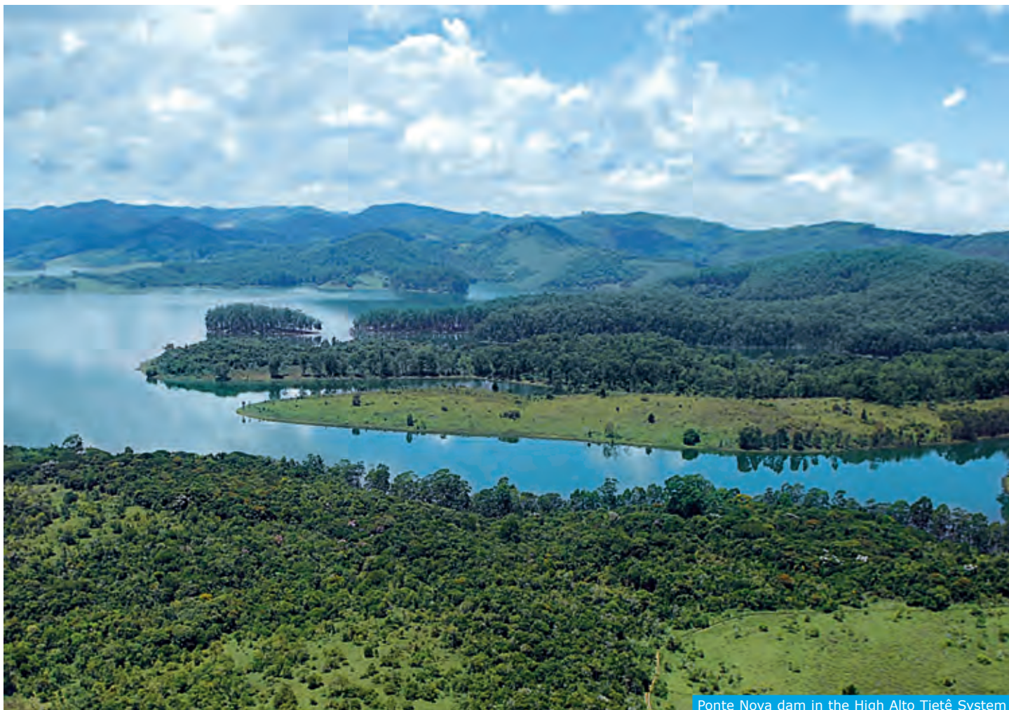
Ponte Nova dam in the High Alto Tietê System
