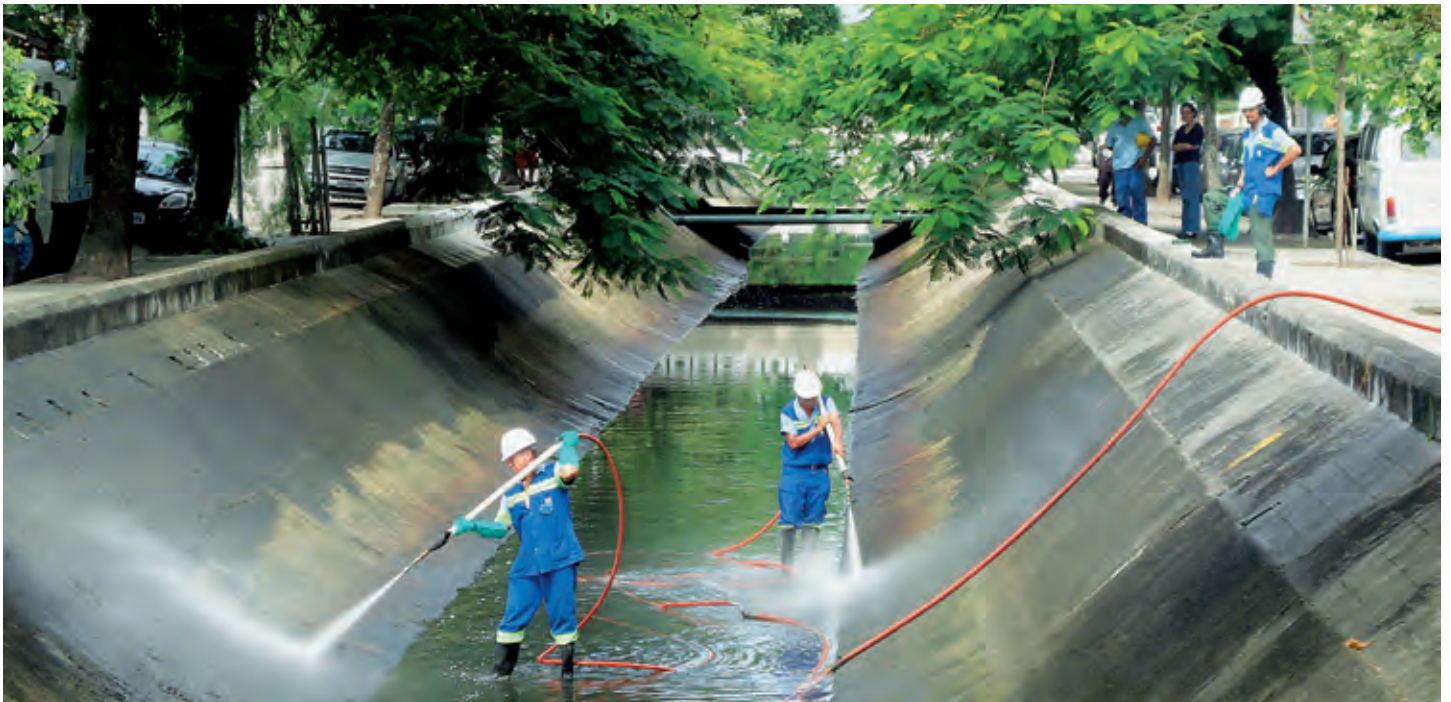
Sabesp employees clean a canal in Santos
