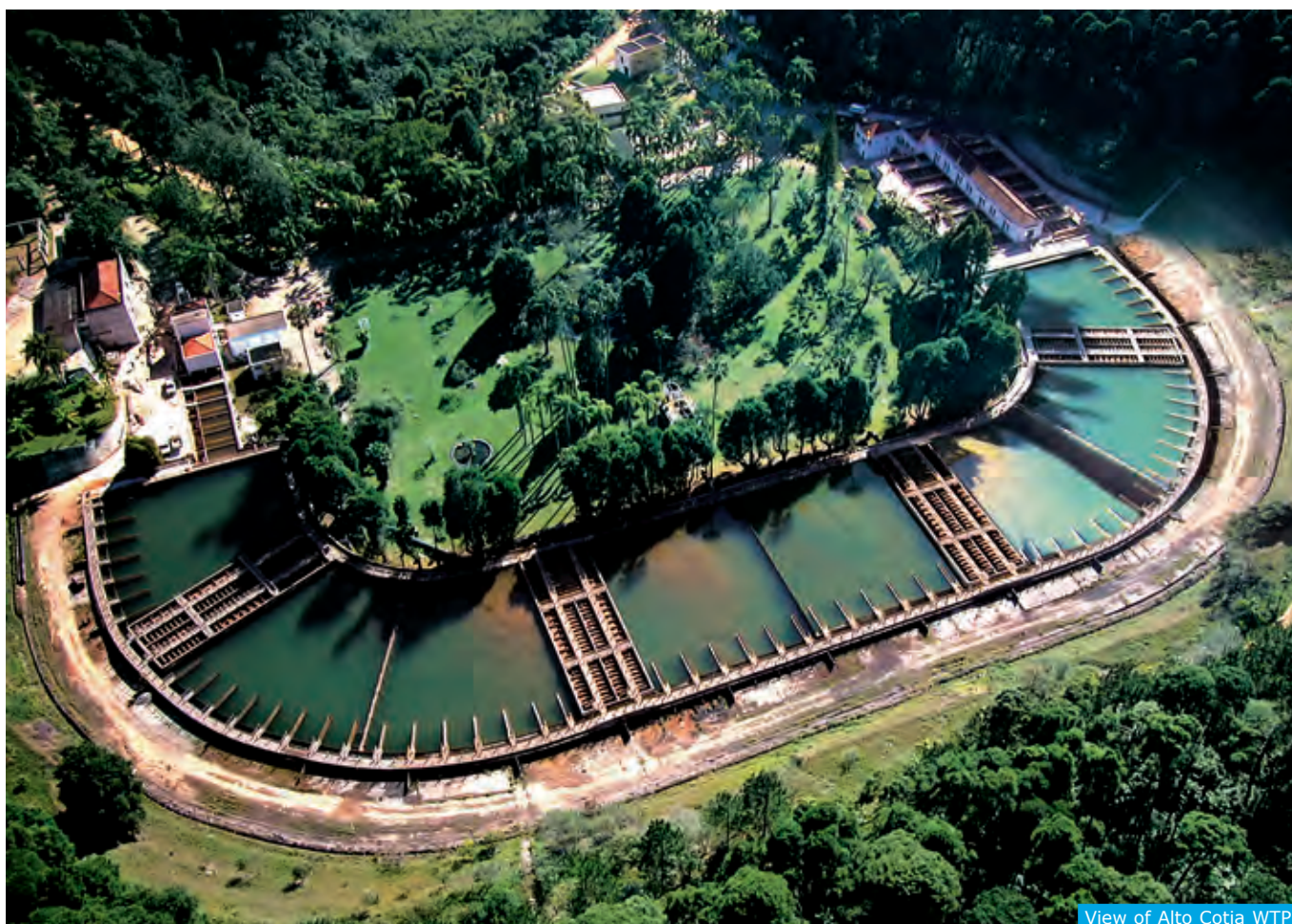
View of Alto Cotia WTP
