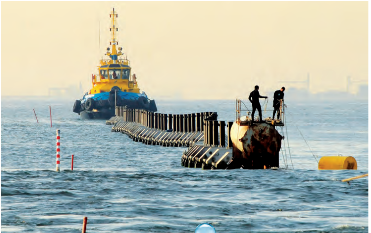
Divers working in the submersion of the Santos sea outfall
