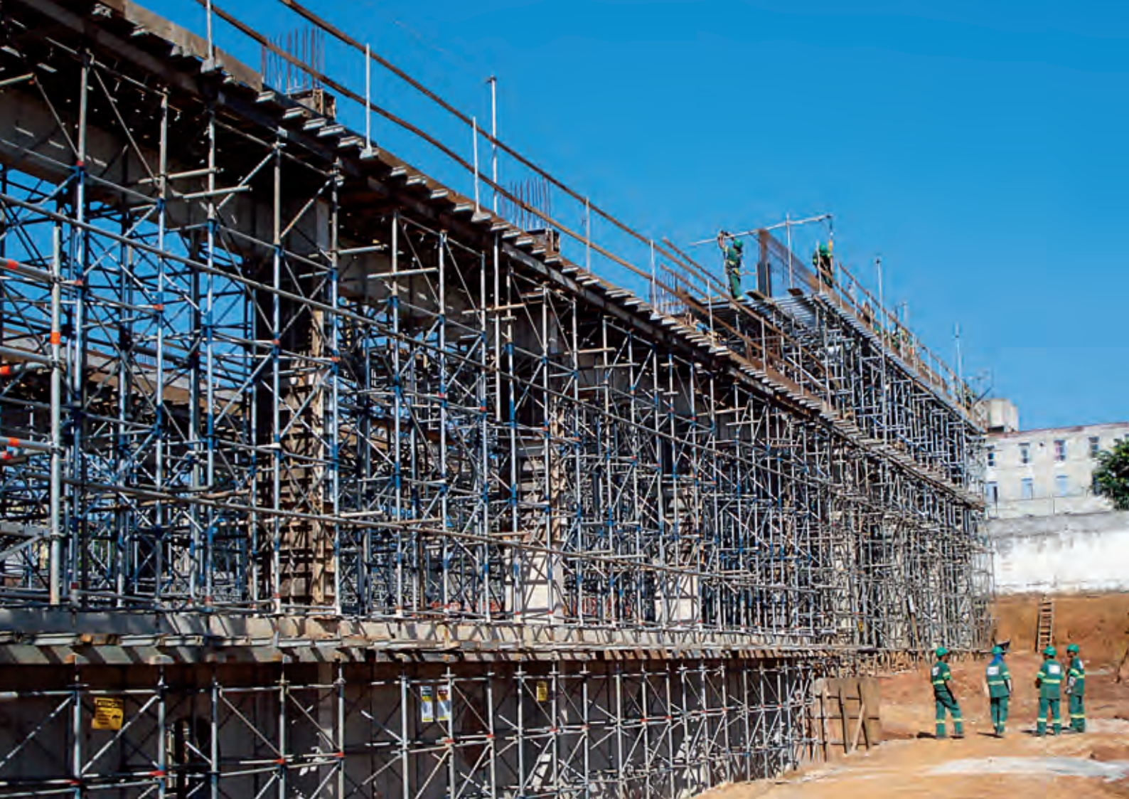
Construction of the Itaquera water lift station
