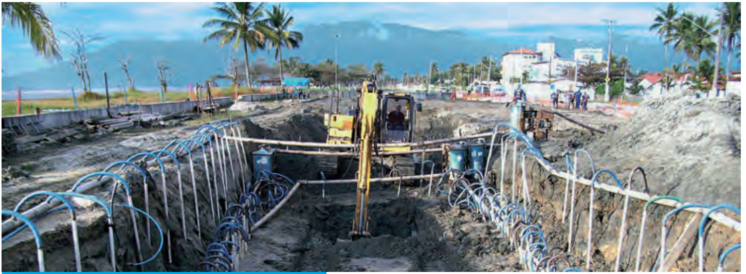
Clean Wave Program construction in Caraguatatuba, North Shore
