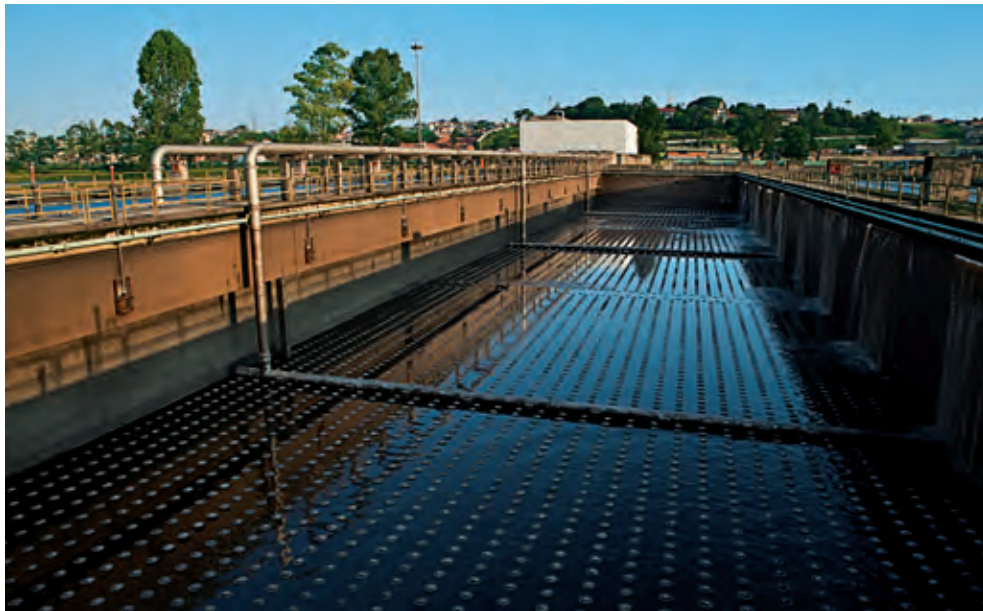
Barueri aeration tank
