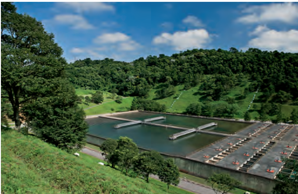
Aerial view of the Guarãú STP
