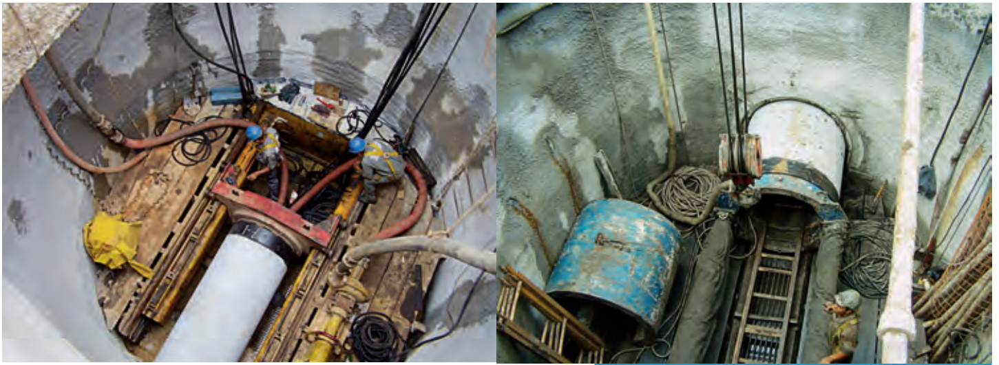
Fixing pipes of the Tietê 15 interceptor, São Paulo East End
