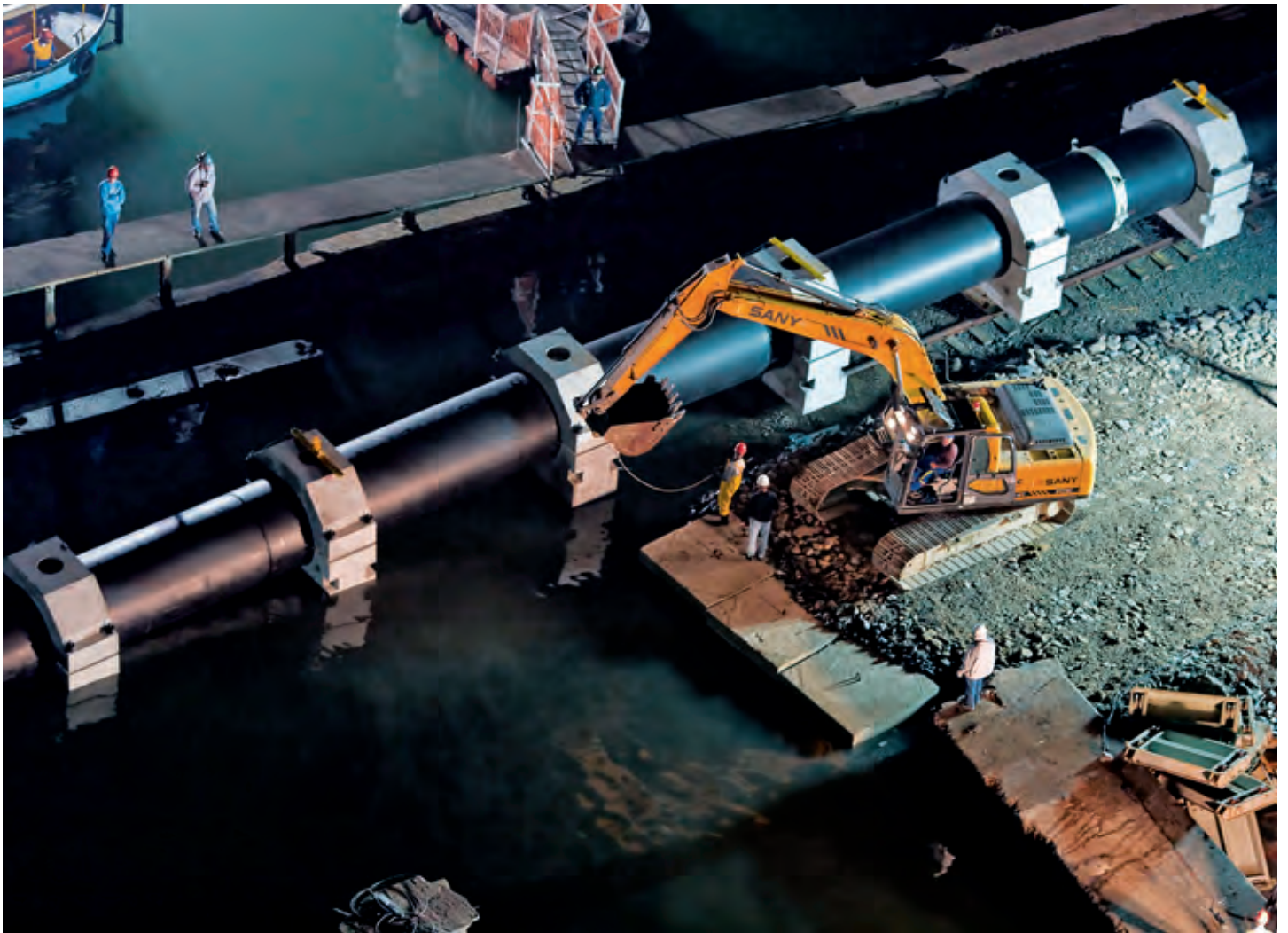
Assembly of a Santos sea outfall span
