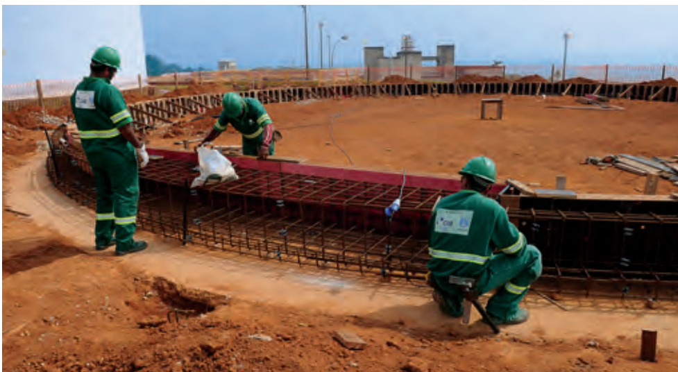
Taiçupeba WTP expansion works
