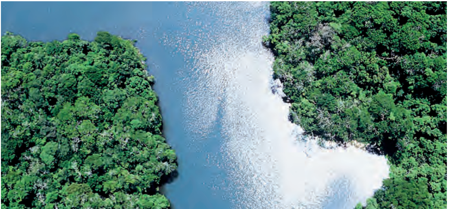
Pedro Beicht dam in the Alto Cotia System
