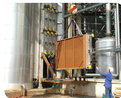
Installation of one of the exchangers
