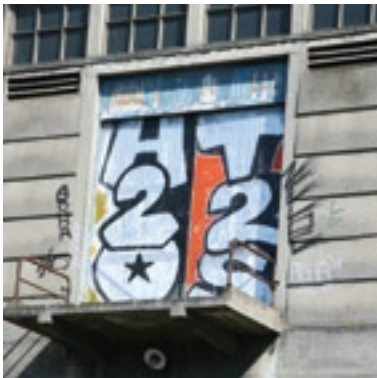
Before: Docks 76 / Rouen prior to renovation and reconstruction
