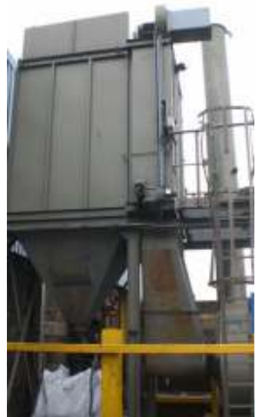
DISA Airmaster dust extraction plant
