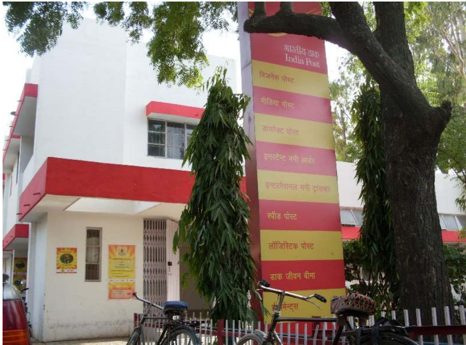
GSK Centre at Salon Sub Post Office, UP
