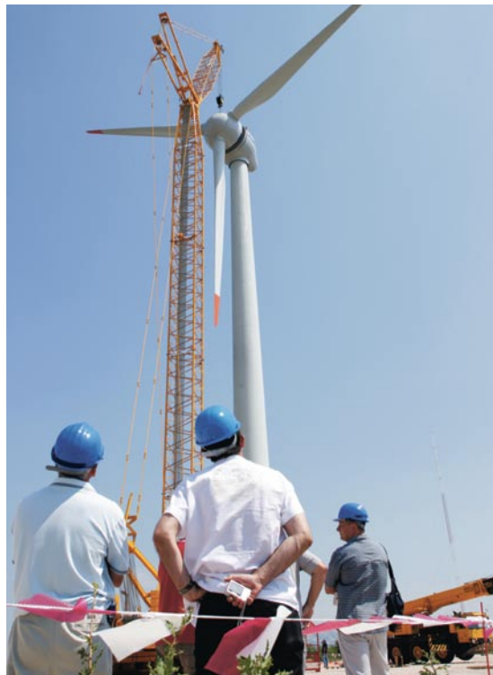
PICTURE 16: WINDTURBINE UNDER CONSTRUCTION
