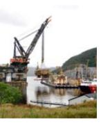
AF has a contract with Shell for the removal, environmental decommissioning and recycling of six platforms on the Indefatigable Field in the British Sector. Parts of the platforms are demolished "piece small" on site, while AF also makes preparations for lifting the remaining modules. These will be transported to the Environmental Base at Vats for further processing and recycling.
