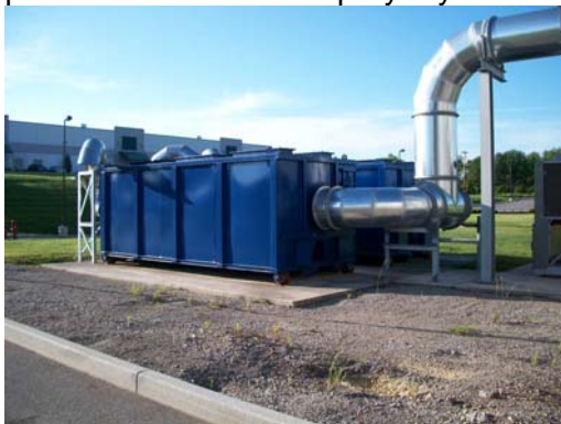
Carbon bed scrubber for odor control
