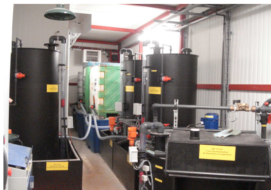
Tanks for the preparation and storage of reagents
