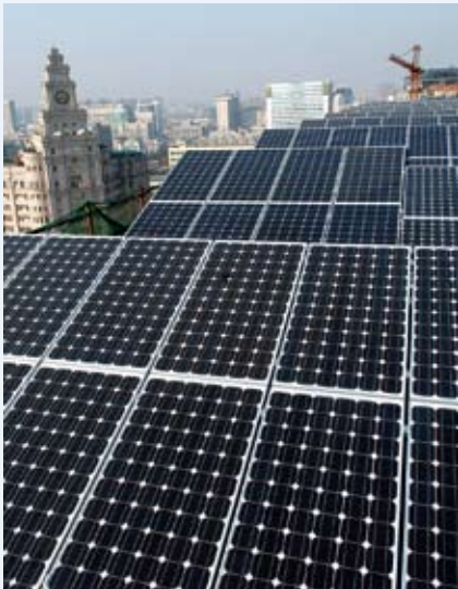
Zhejiang Electric Power Company's 250kW grid-connected rooftop solar PV pilot power station
