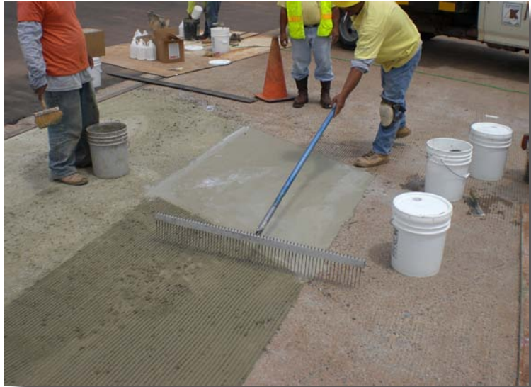
SINAK Relay Resurfacer being used as a low VOC alternative for highway patching.
