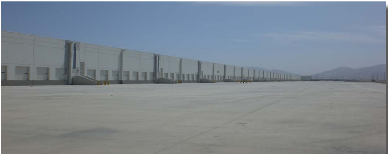
SINAK S-102 used in place of water cure to save millions of liters of water in Southern California.
