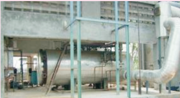
Waste heat recovery boiler
