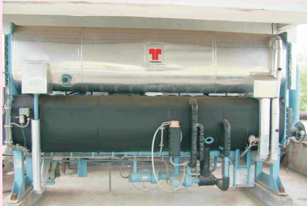
90 TR CHW Plant from CPP flue Gas heat
