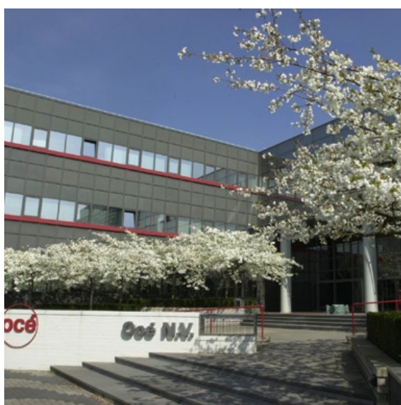
Océ headquarters in Venlo, The Netherlands.
