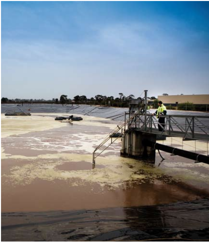
Wolf Blass winery wastewater treatment facility.
