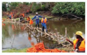
Laying a seismic cable across a river at Gabon
