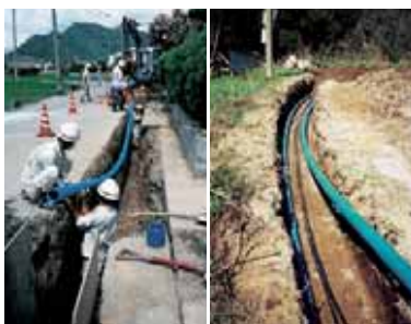
Installation of high-performance pipe materials with superior earthquake resistance and ease of installation
