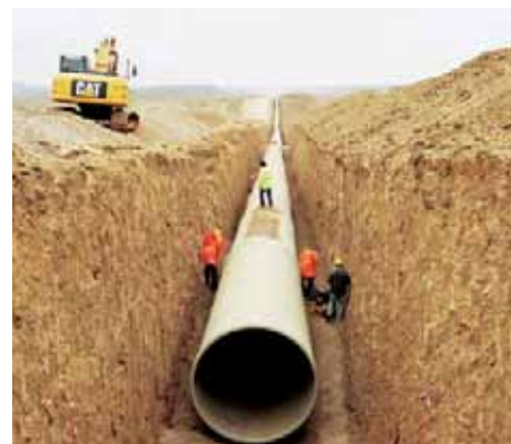
Aqueduct construction in Azerbaijan (reinforced plastic pipe)
