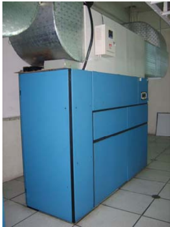
Energy-saving heat exchange device installed on the air-conditioner in the equipment room—indoors
