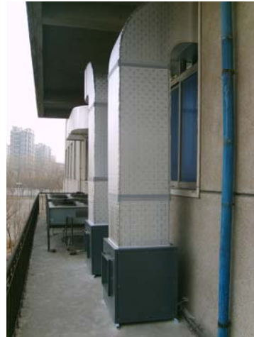
Energy-saving heat exchange device installed on the air-conditioner in the equipment room—outdoors
