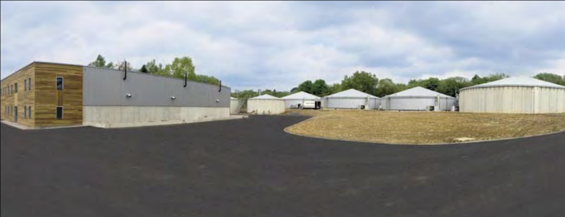
► The newly constructed bio-methane cogeneration facility in Libramont (Belgium), which is scheduled for operation in September 2009.
