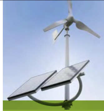
► Solar panels with windmill stand-by generator, Pudong (China).
