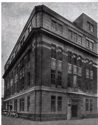
Sumitomo Building Annex, where Nippon Kensetsu Sangyo's head office was located
