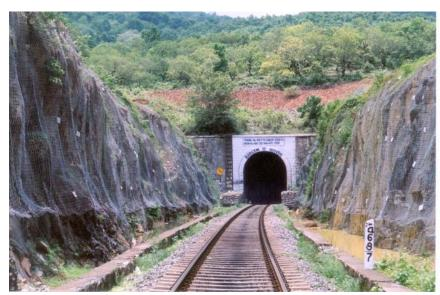
Boulder Netting and Geo-safety works have been carried out on a large scale throughout Konkan Railway route strengthen the cuttings and to protect the environment.
