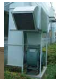
Exhaust vent with a noise reduction cover
