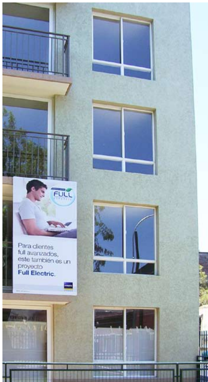
Edificio Full Electric.
