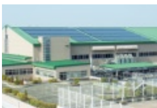
Rooftop solar power generation system at Hakata Brewery
