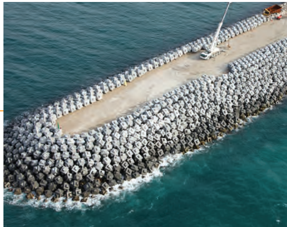
Use of the cubipod in the harbor wall work at Langosteira port, in A Coruña, Spain.
