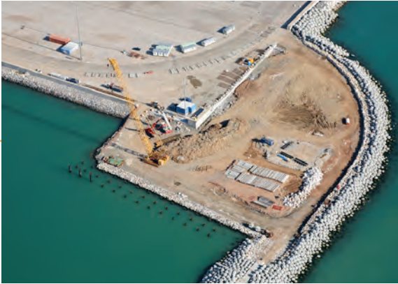
Breakwater built with cubipods at the Port of Malaga.
