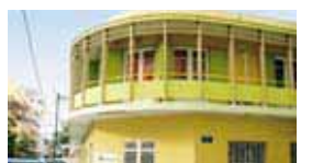
GTZ Office, Dakar, Senegal
