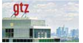
GTZ Head Office, Eschborn near Frankfurt am Main
