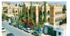
GTZ Office, Sana'a, Yemen
