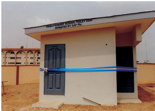
Newly constructed Four-way toilet for pupils and teachers of Ogba Primary School, Lagos
