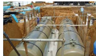
Renovations installing double-walled tanks
