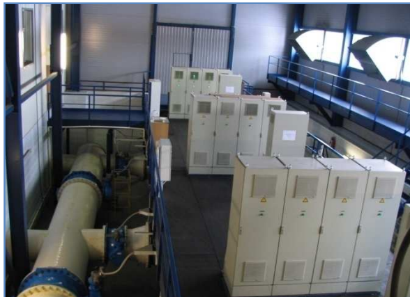
Second stage – ultraviolet disinfection
