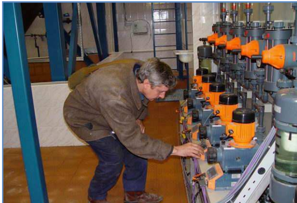
First stage – chlorination and ammonization with use of safety chemical agents: sodium hypochlorite and ammonium sulfate
