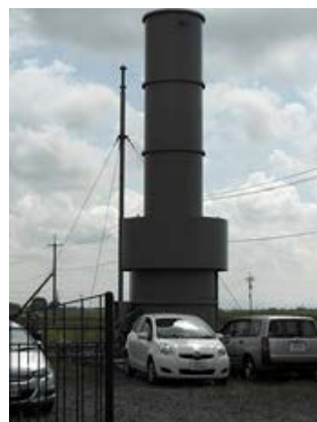
A ground flare system at the facility for collection of newly extracted oil at the Akita District Office
