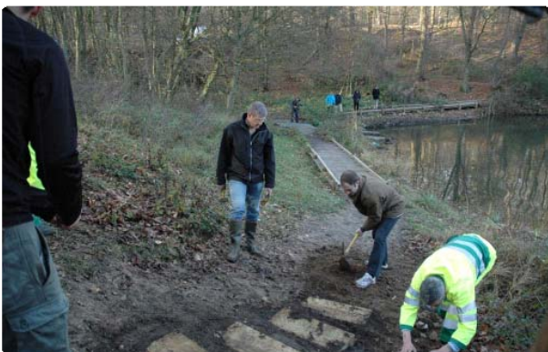
Building the staircase to improve public access
