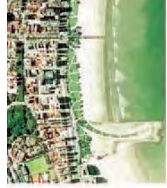
EPC Santos / São Vicente aerial view
