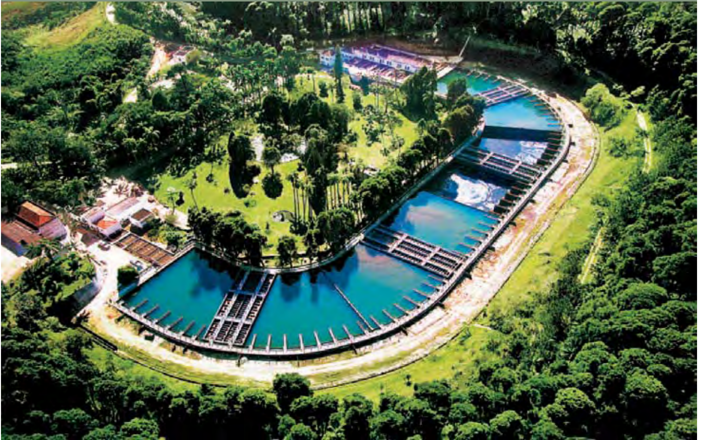
High Cotia Water Treatment Station.
