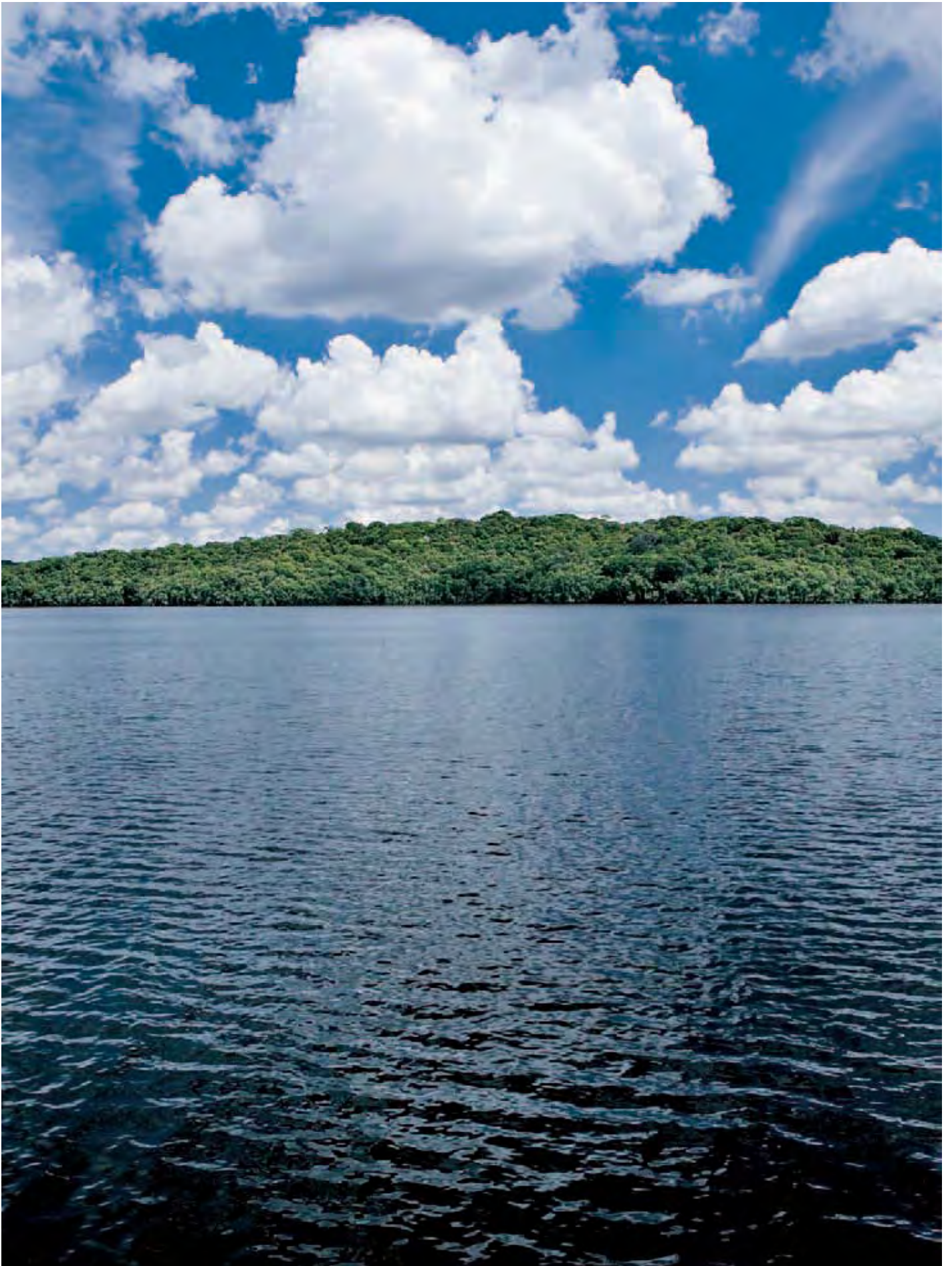
Dam serving the High Cotia Water Treatment Station.
