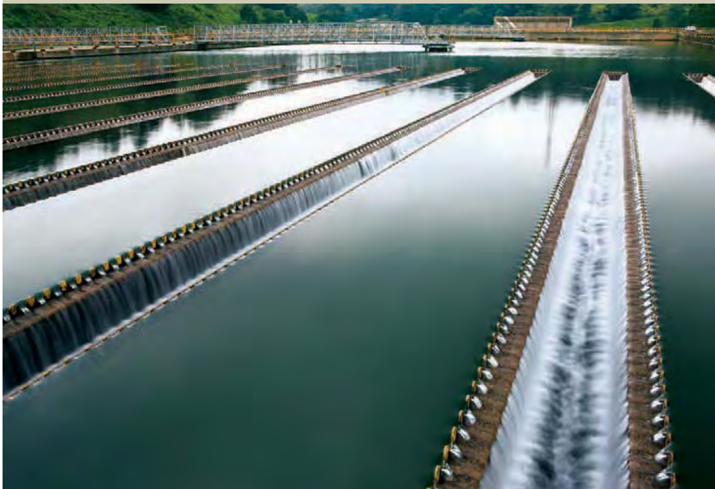
High Cotia Water Treatment Station.
