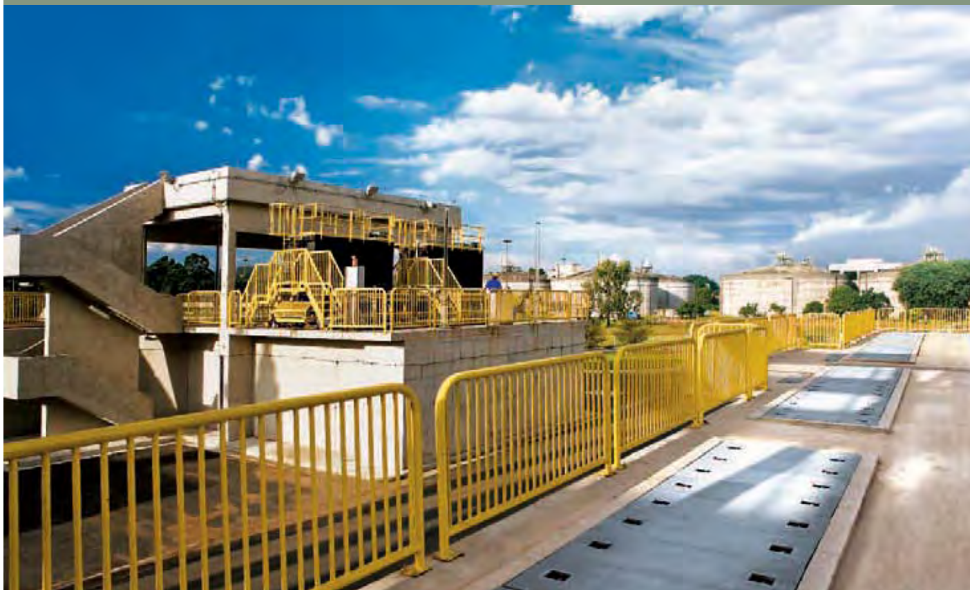
Barueri Sewage Treatment Station.
