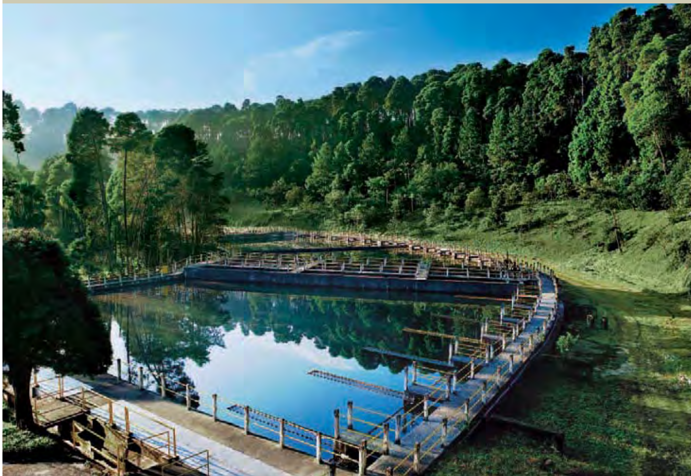
High Cotia Water Treatment Station.
