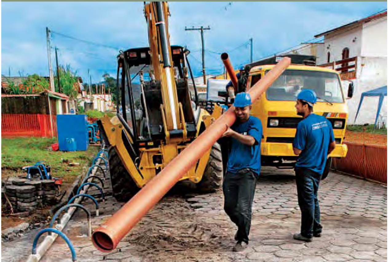
Construction of Clean Wave Program, in Baixada Santista.
