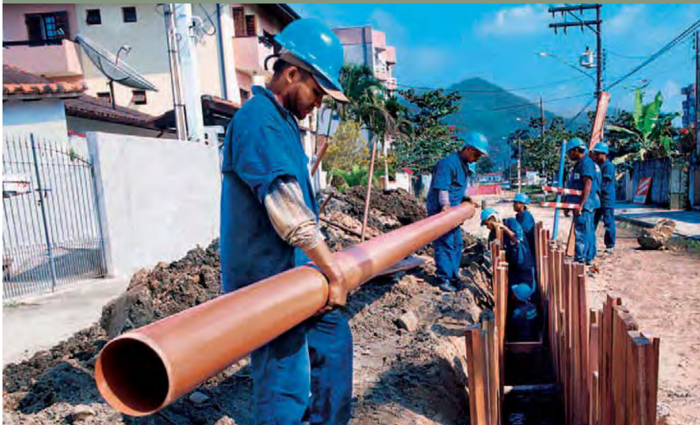
Sewage Connection in Bertoga.
