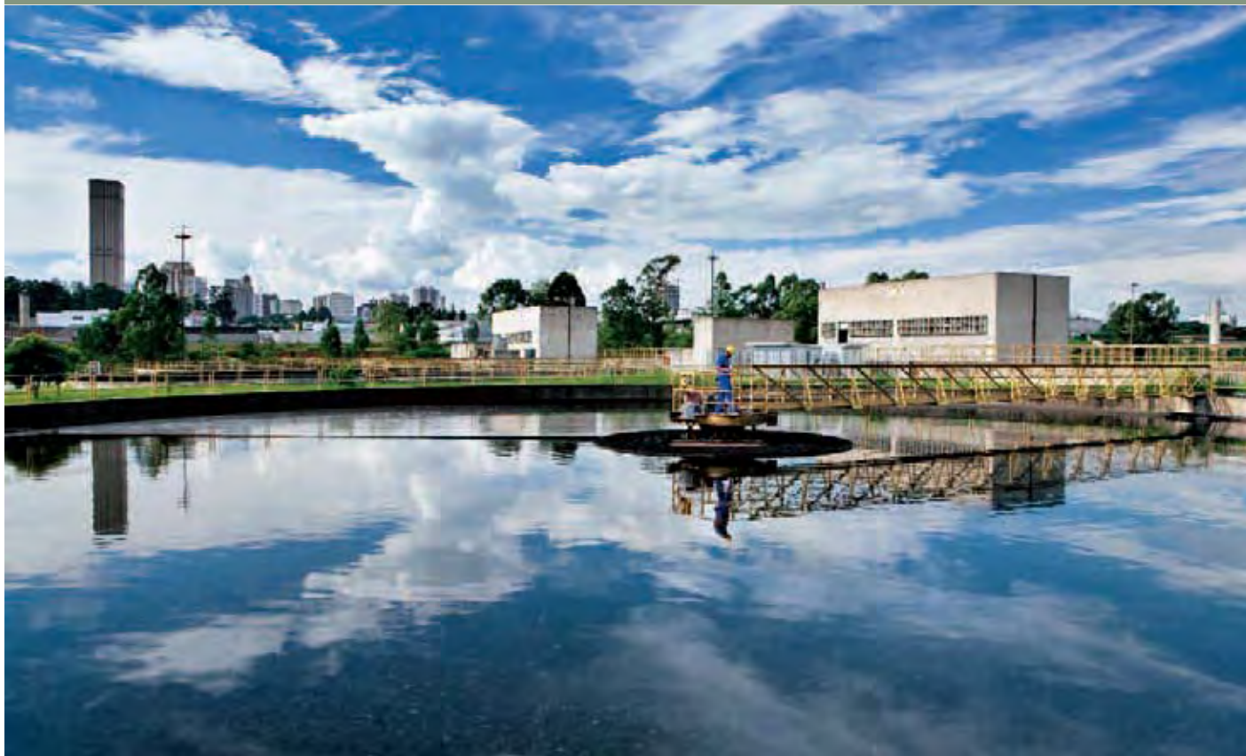
Barueri Sewage Treatment Station.
