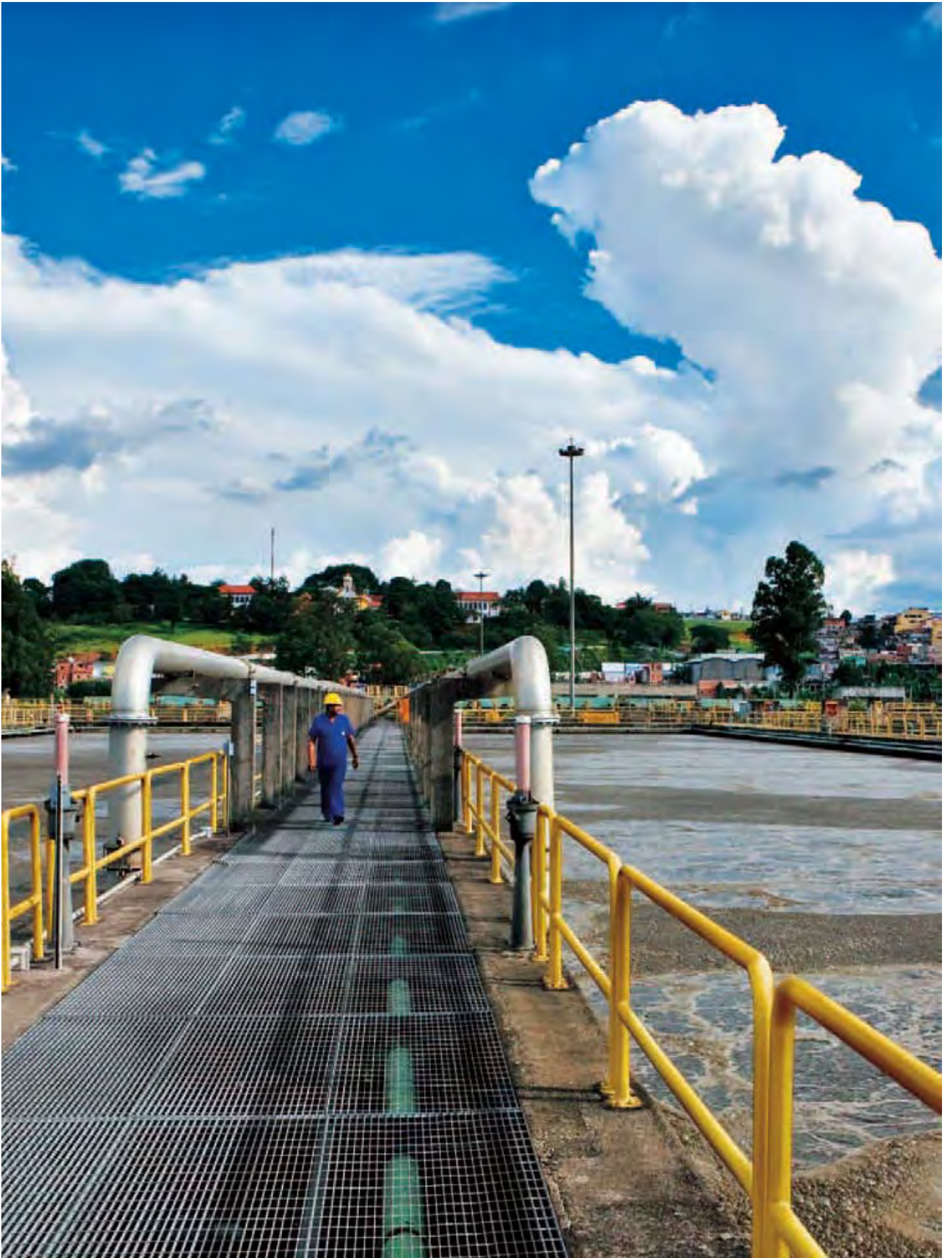
Barueri Sewage Treatment Station.
