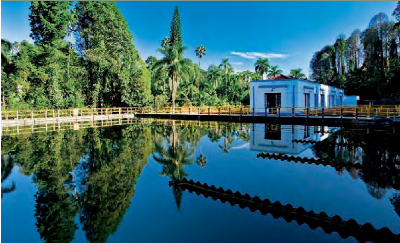
High Cotia Water Treatment Station.
