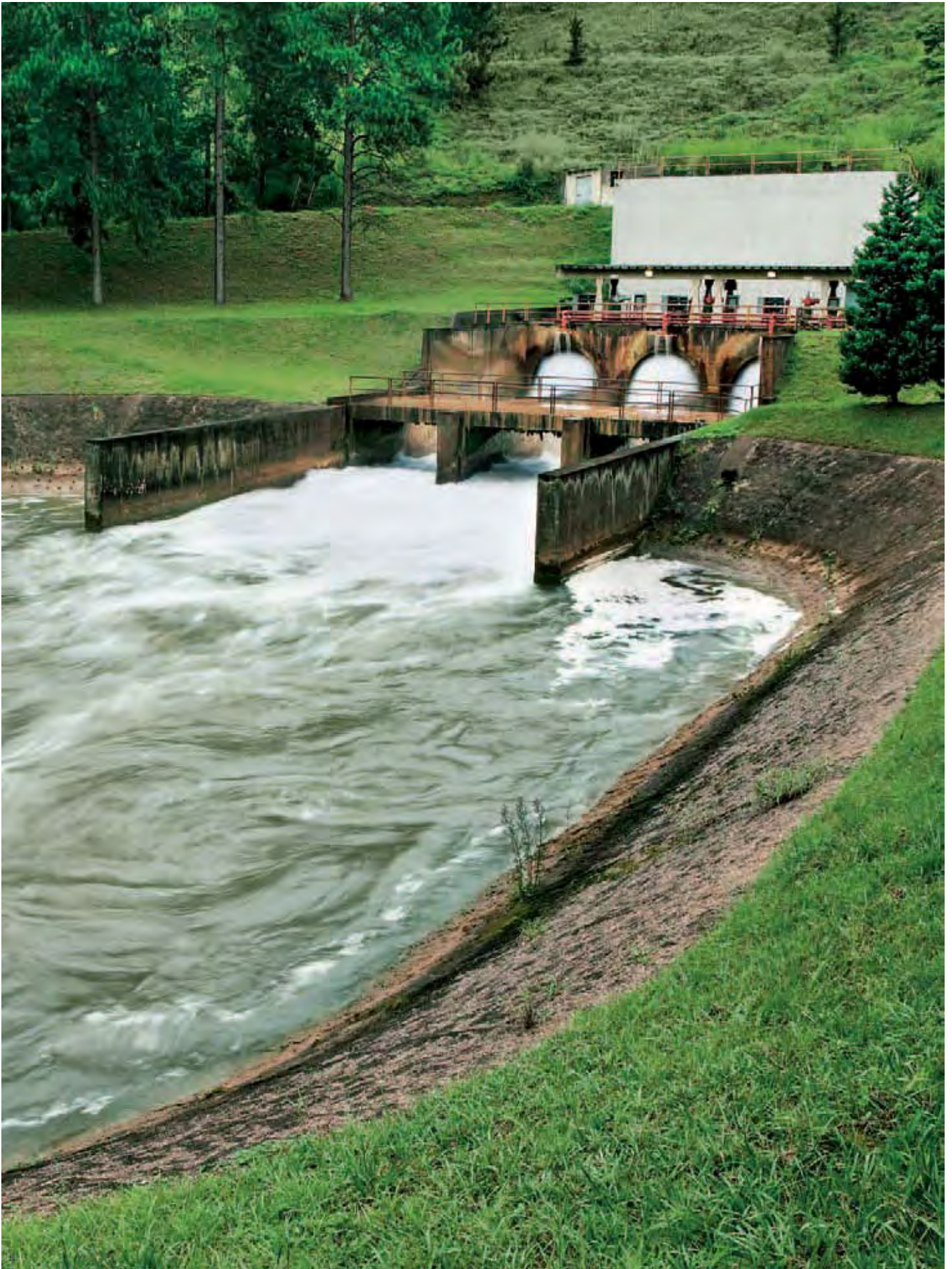
Arrival of the water at the Guarú Treatment Station, in São Paulo.
