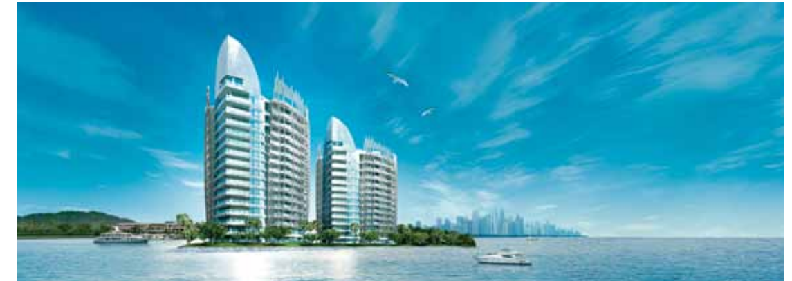
THE OCEANFRONT @ SENTOSA COVE – Residents at this exclusive waterfront condominium can expect to save up to S$1,000 per apartment per year from the energy-efficient air-conditioners. It is the first condominium in Singapore to incorporate a system to recycle water from apartment bathtubs, showers and wash basins for flushing of clubhouse toilets and irrigation of landscape.
