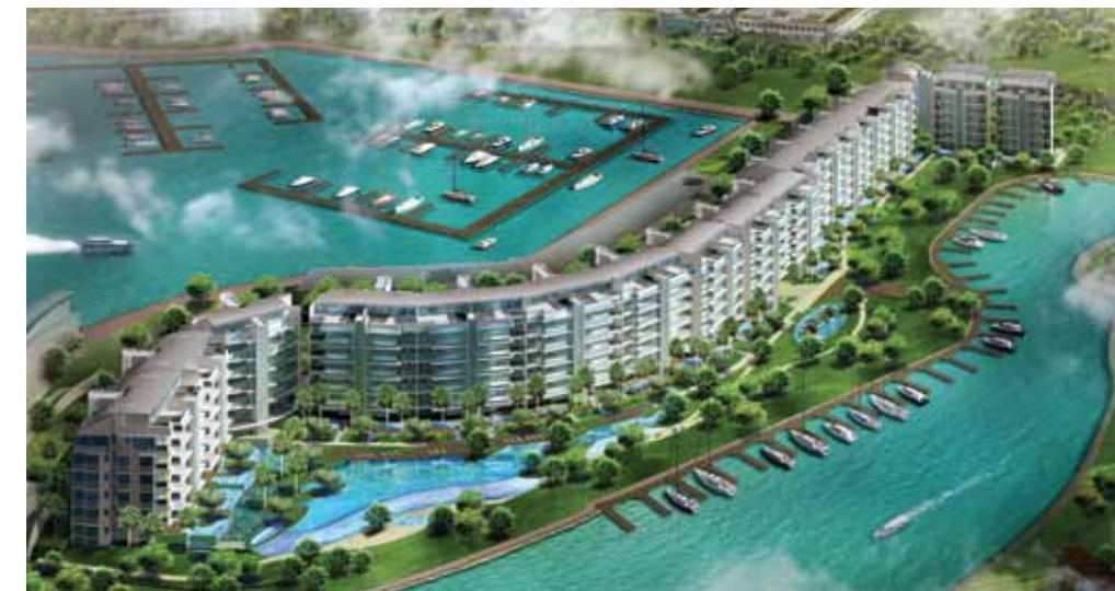
QUAYSIDE ISLE COLLECTION AT SENTOSA COVE (RESIDENTIAL) – Residents can enjoy energy savings of up to S$2,500 per apartment annually from the energy efficient green features incorporated within their homes.
