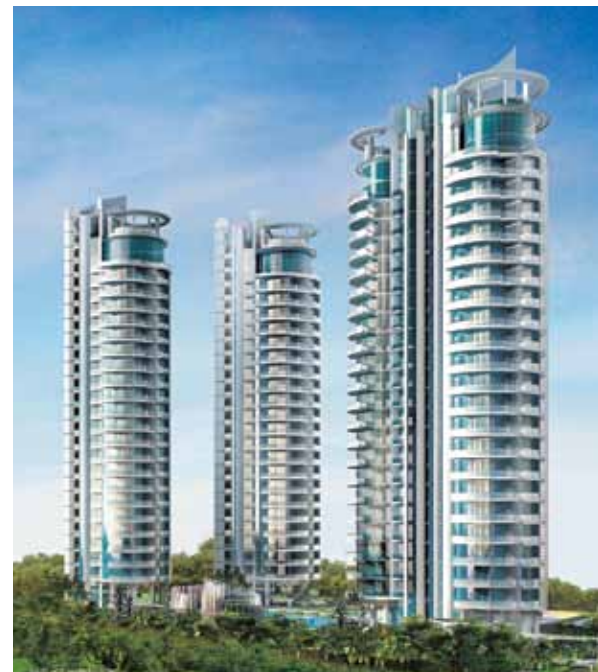
CLIVEDEN AT GRANGE – Exceptional “Green” clubhouse with an innovative photocatalyst coating with water film system to cool down the internal and external environment. The various energy-efficient features help reduce energy costs by approximately over S$400,000 per year.
