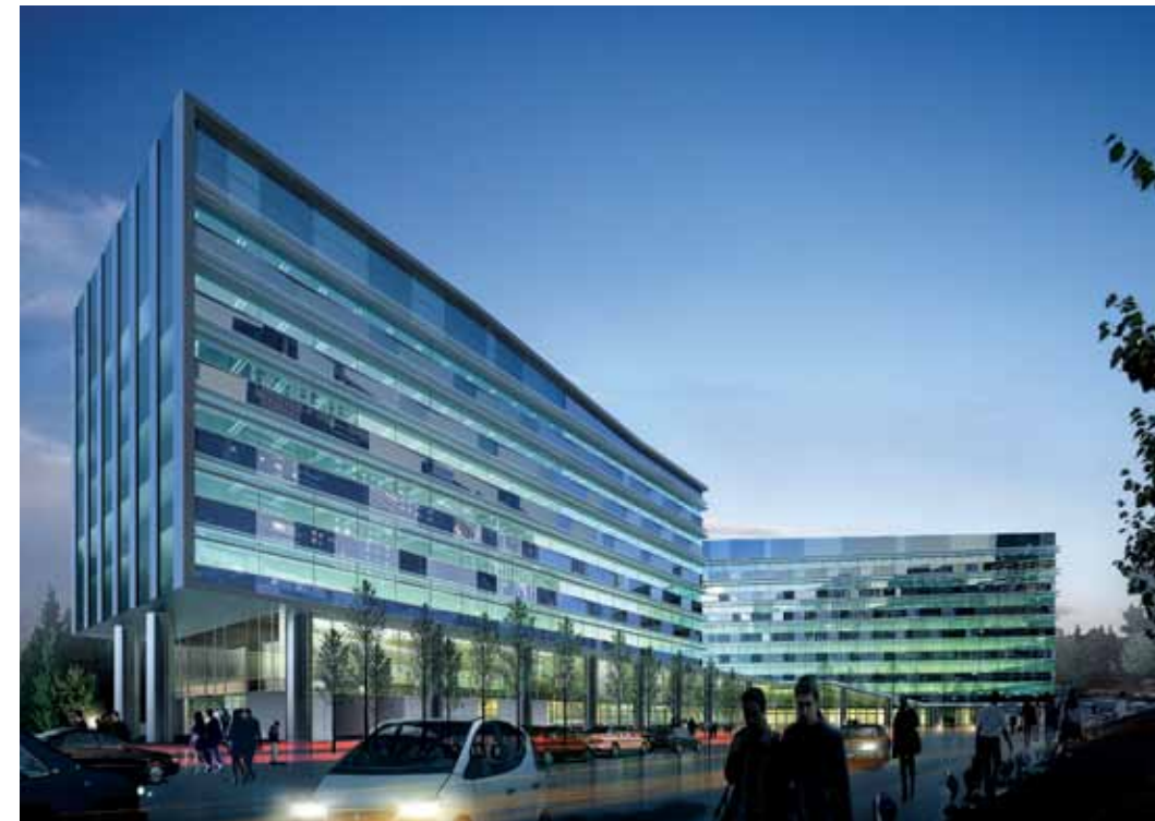
7 & 9 TAMPINES GRANDE – A state-of-the-art new generation green office building with invested approximately 4% of the construction cost incorporating green features in the development's green features. The 300,000 square feet building comprising twin eight-storey office blocks was constructed with eco-friendly materials and integrated with numerous green features.
