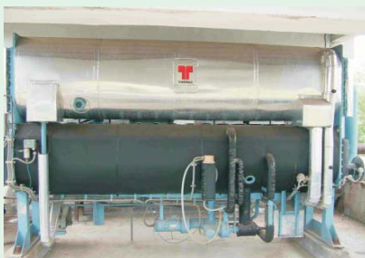
90 TR CHW Plant from CPP flue Gas heat
