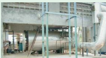
Waste heat recovery boiler
