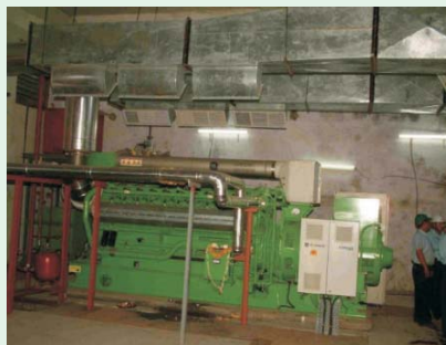
1MW CO - GEN Power Plant (CPP) on Gas
