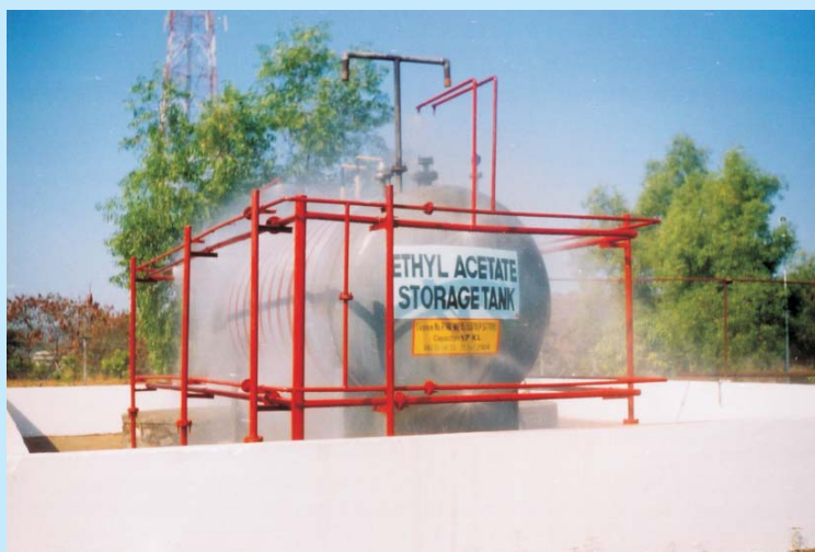
Storage Tank emergency water spray
