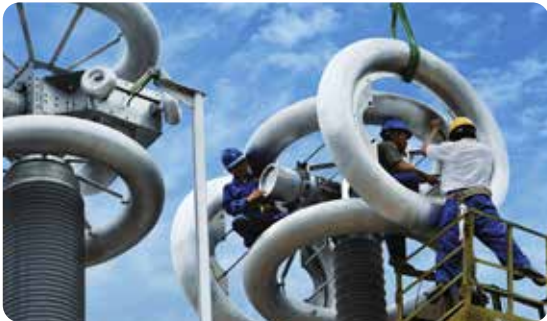
▲ Staff installing current equalizer at Suidong converter station for the ±800 kV UHVDC Yunnan-Guangdong project.
