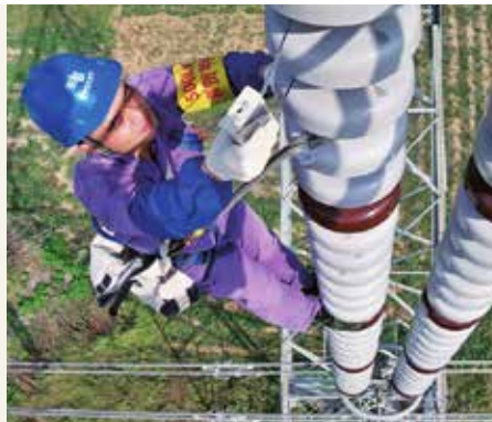
Left: Staff on duty are testing the temperature of equipment in operation.
