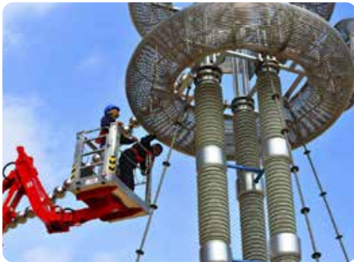
▲ The engineers are carefully examining the grading ring of ultra-high voltage experimental equipment.
