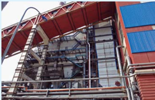
Bag-type precipitation and flue gas denitration facility
