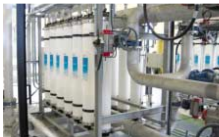
▶ Waste water treatment facility
