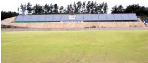
▶ Taeon solar power plant
