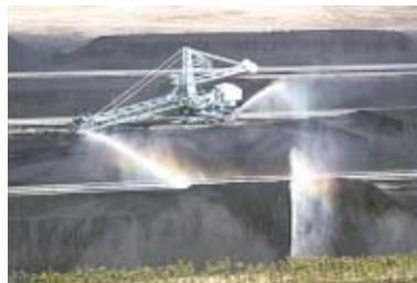
► Water sprinkling facility
