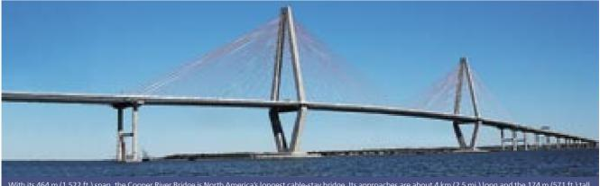
With its 464 m (1,522 ft.) span, the Cooper River Bridge is North America's longest cable-stay bridge. Its approaches are about 4 km (2.5 mi.) long and the 174 m (571 ft.) tall towers, or pylons, have given neighboring Charleston and Mount Pleasant, South Carolina a new landmark.
