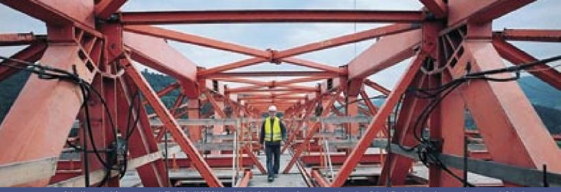
Poland has major infrastructure needs. The 600 m (1,968 ft.) long Milówka Bridge is part of an expressway in southern Poland. Skanska is the only construction company in Poland with access to the rolling scaffolding shown here, used in formwork of permanent bridge structures. Skanska is also responsible for building 90 km (56 mi.) of the A1 highway in northern Poland as part of a public-private partnership.
