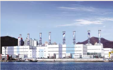
Metropolitan Areas' Environment-Friendly Power Plant Busan Combined Cycle Power Site Div. (759-8, Gamcheon 1 dong, Saha-ku, Busan) Fuel used: LNG Capacity: 1,800 MW(G/T 150 X 8units, S/T 150 X 4units)
