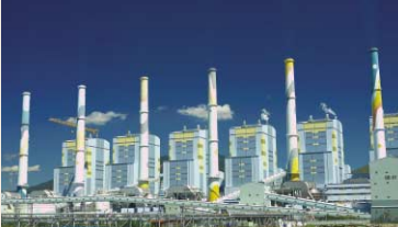
The Epitome of Korea's Standard Coal Thermal Power Plant Hadong Thermal Power Site Div. (310, Gaduk-ri, Geumsung-myun, Hadong-kun, Kyungsangnam-do) Fuel used: Bituminous coal Capacity: 3,000MW(500 X 6units) ※1,000MW(500 X 2units under construction)
