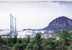
Center of Power Supply in Clean Jeju Area Namjeju Thermal Power Plant (610, Hwasoon-ri, Anduk-myun, Seogwipo-si, Jeju) Fuel used: Heavy oil Capacity: 240 MW(Machine power 100 X 2units, Internal combustion 10 X 4units)
