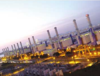
Motive Power for Development of Metropolitan Industry Shinincheon Combined Cycle Power Site Div. (674-13, Kyungseo-dong, Seo-ku, Incheon) Fuel used: LNG Capacity: 1,800 MW(G/T 150 X 8units, S/T 150 X 4units)
