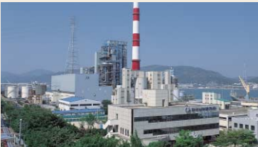
Driving Force of Economic Development in Ulsan Area Youngnam Thermal Power Plant (29, Maeam-dong, Nam-ku, Ulsan) Fuel used: Heavy oil Capacity: 400 MW(200 X 2units)
