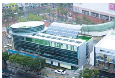
Additional photovoltaic power generator
