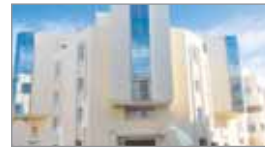
GTZ Office, Tunis, Tunisia
