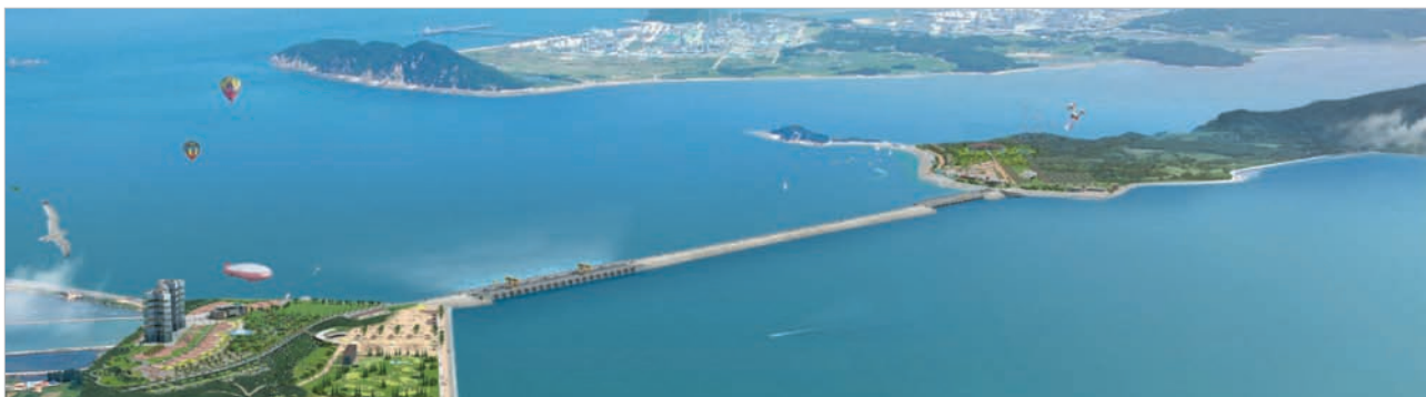
▲ Garolim Tidal Power Plant
