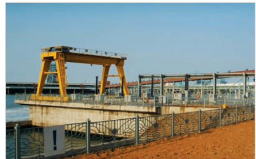
▲ Taean Small Hydro Power Plant
