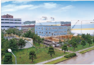
▲ Wastewater treatment facilities
