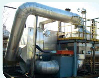
3,000Nm 3 /h sewage farm waste gas catalytic combustion processing installation
