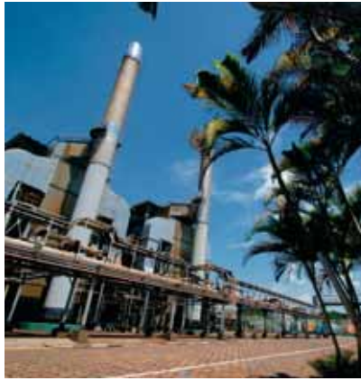
1 Site operator, Acetow, Freiburg (Germany)
