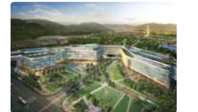
Sejong City Government Office (May 2012/Eco-friendly Structure Pre-certification)
