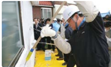
House Repair of Hope
