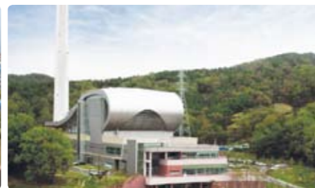
Chungju Area Incineration Plant
