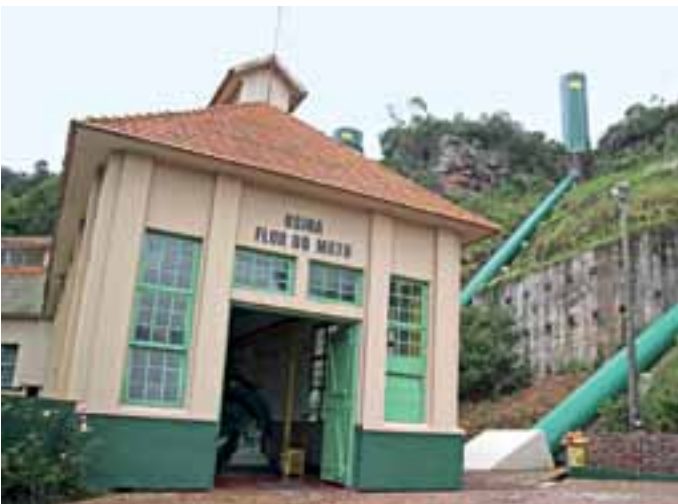
Flor do Mato Plant: In 2012, the hydroelectric power station was responsible for 10.80% of the energy consumed by IRANI
