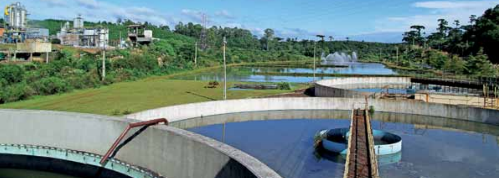
Wastewater Treatment Plant: strict control and management of water resources
