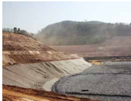
— Essencis – Landfill – Caieiras, SP — Construction of water supply system – Irerê, BA
