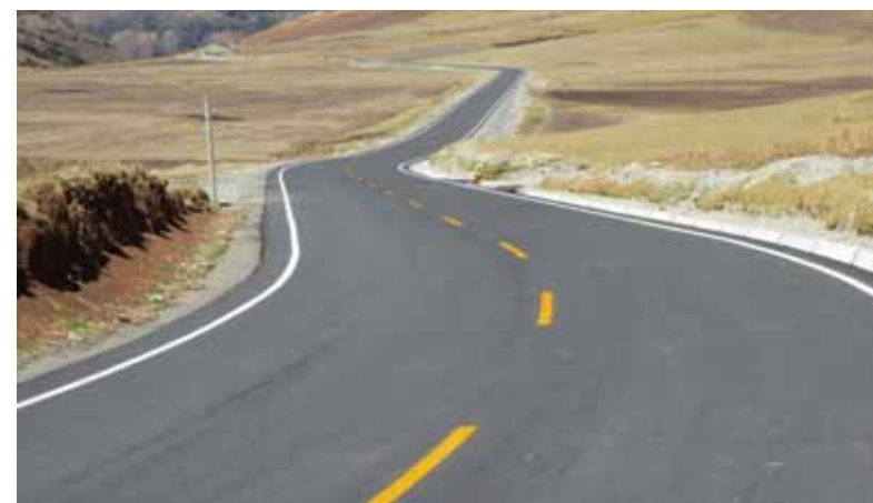
Ayacucho Highway - Abancay, Peru
