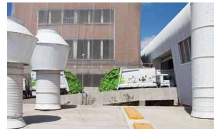
Loga – Transfer Facilities – São Paulo, SP
